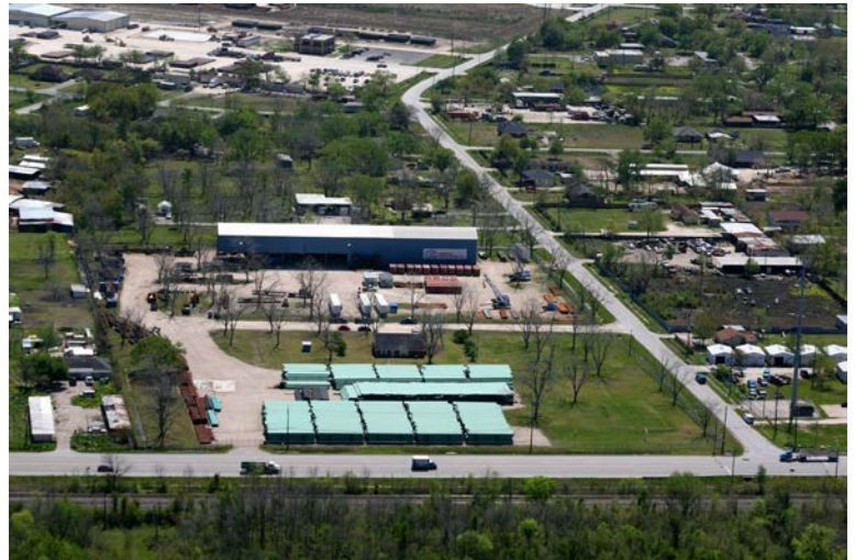
Houston Fabrication & Yard
